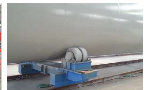
Sandblasting and painting
