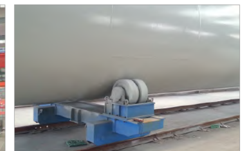
Sandblasting and painting
