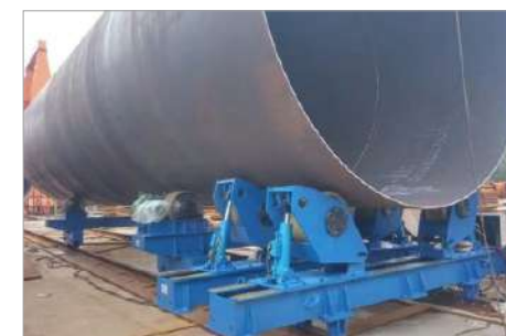
Flange fit-up & welding
